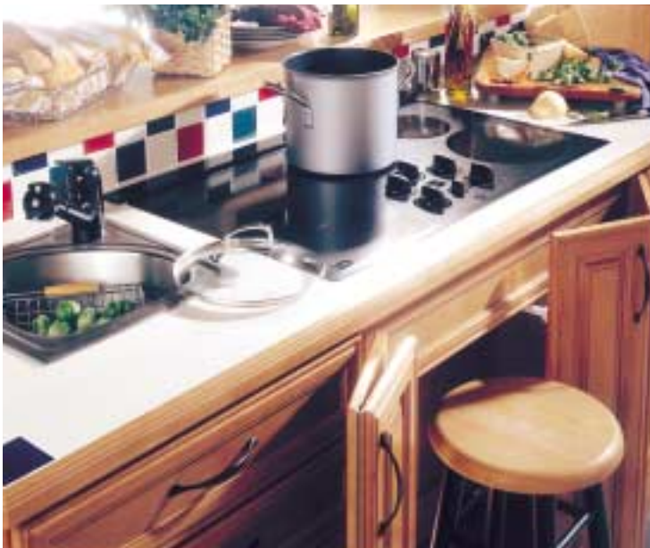
The open knee space under this cooktop provides a comfortable working area.
