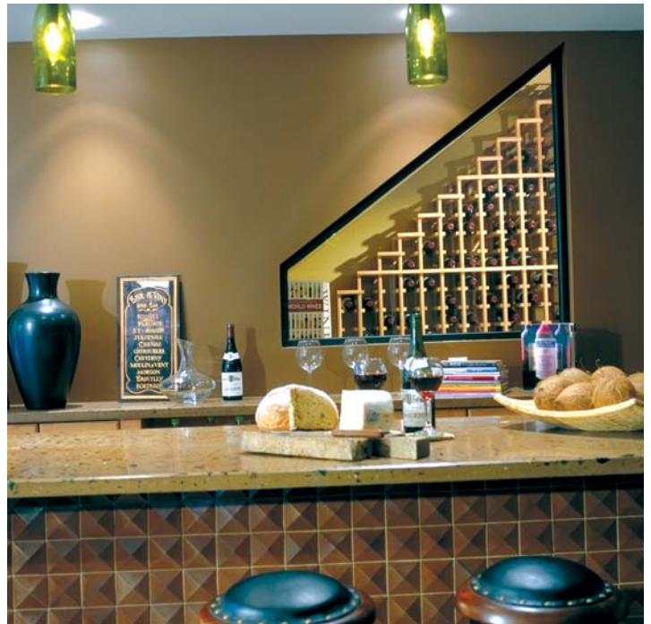
The large triangular window behind the bar permits views inside the wine and beverage cooler. The wine theme is continued in the light fixtures and in the countertop made from concrete mixed with pieces of broken wine bottles.
